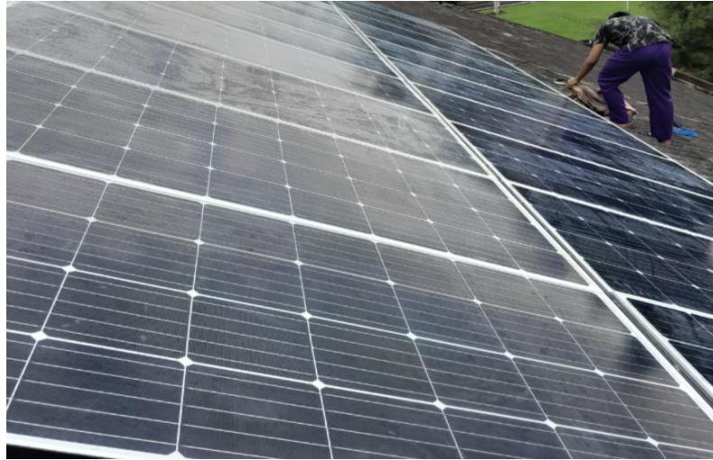
Figure 1. Solar panel research equipment
