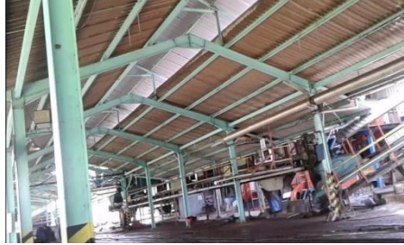
Figure 5. Sterilizer Station Roof
