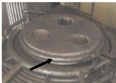
Figure 3. Electric arc furnace small cap bearing pipe
