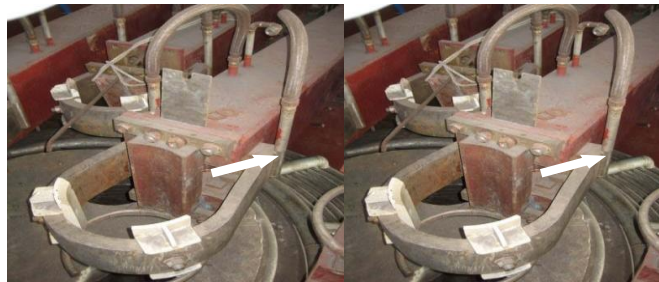
Figure 5. Electric arc furnace electrode support cooling pipe
